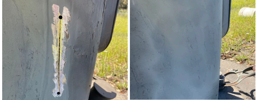
Figure 17: Repair of overhead sign structure hairline crack (before & after).
